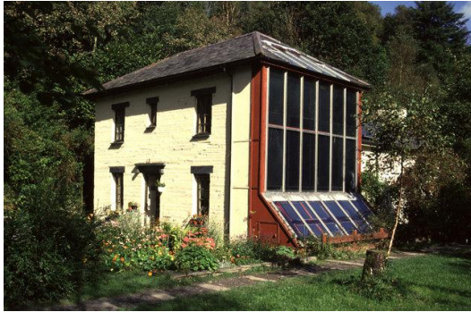
Figure 1: Allen, C (1993) House with solar wall. Centre for Alternative Technology, Wales [Online image] [Accessed on ...]
